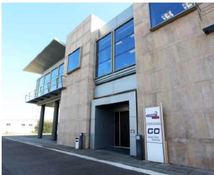
Entrance to the offices of the new premises.
