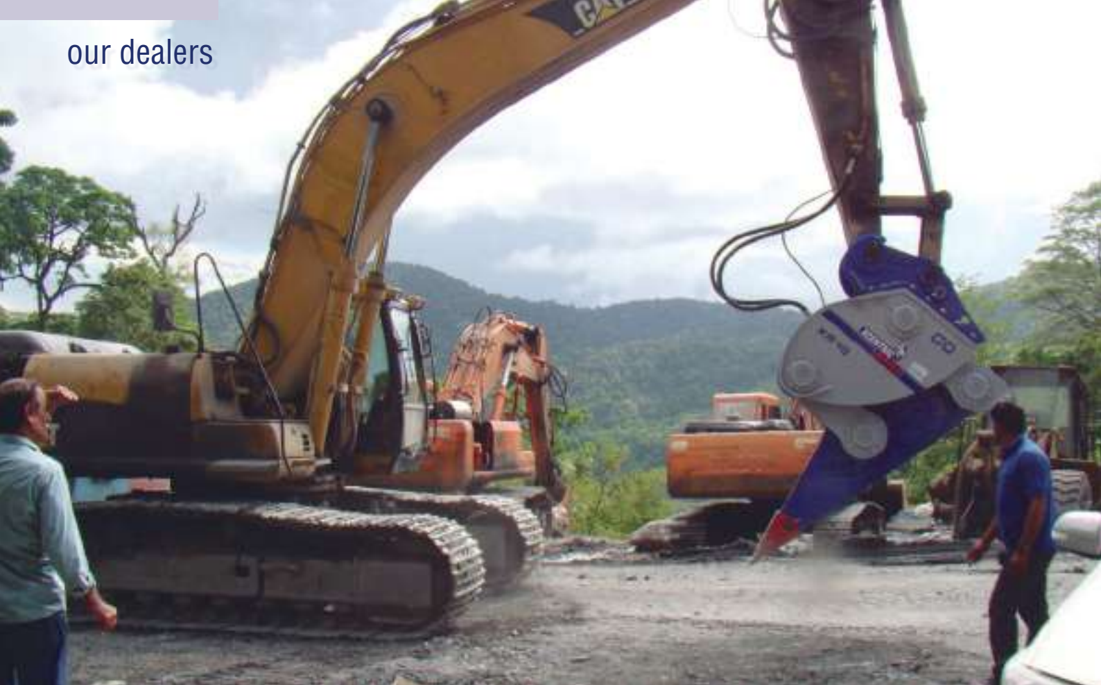
Xcentric Ripper XR40 working in Trinidad & Tobago.
