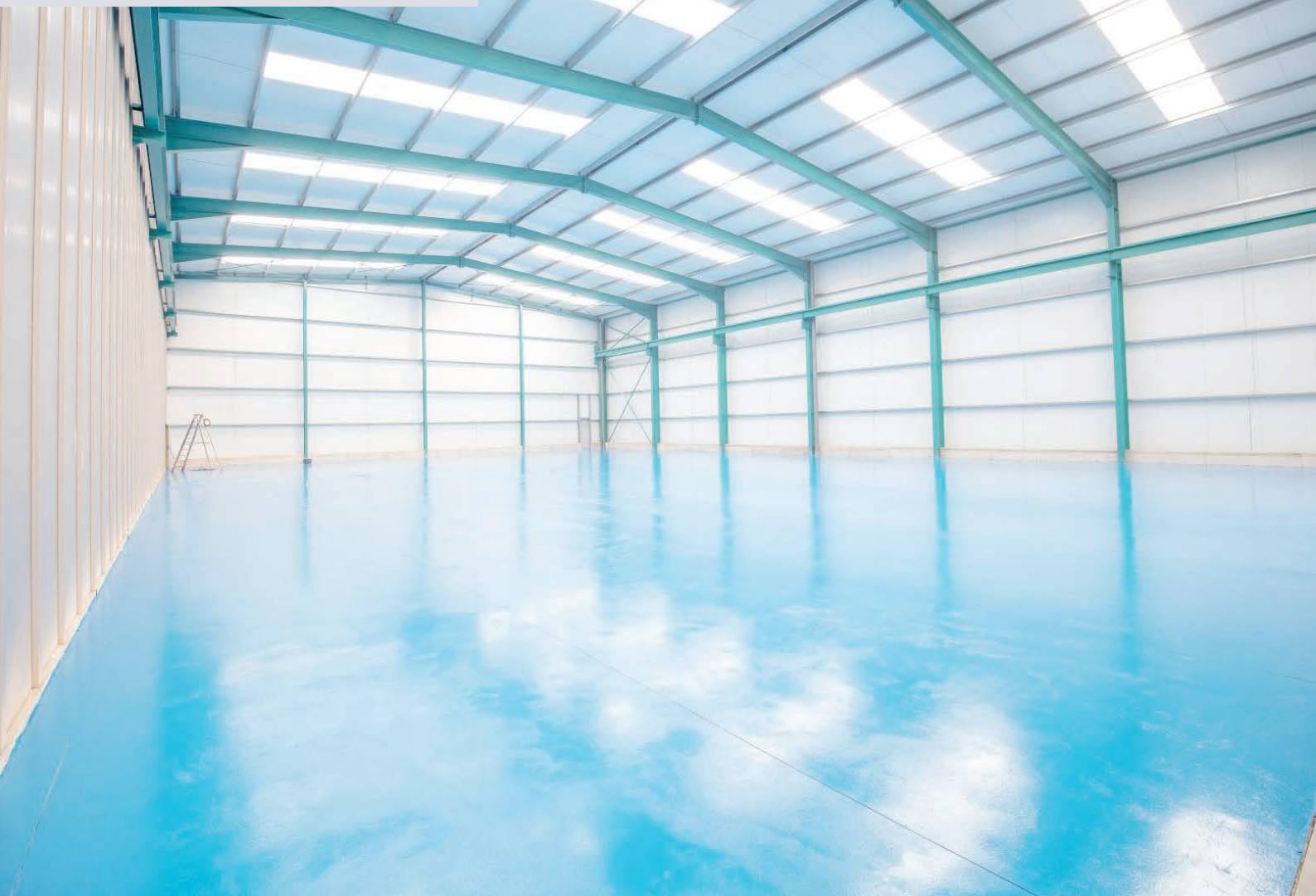
The new pavilion at the Xcentric factory in Vitoria-Gasteiz.
